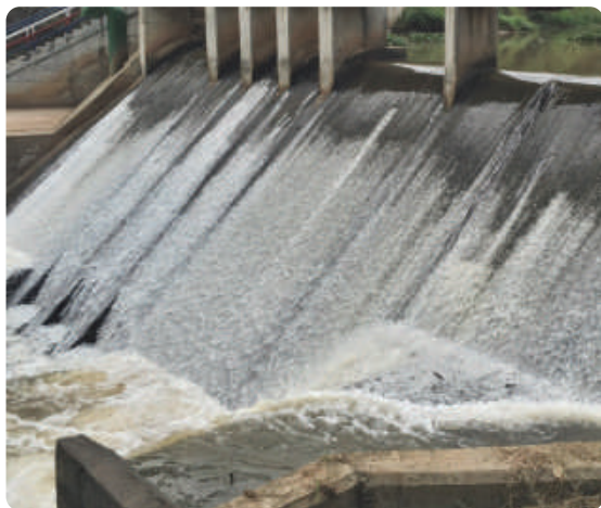
Fig 15.7 Mukungwa hydroelectric power generation
