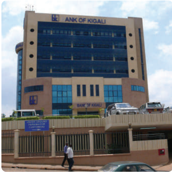
Fig 10.10 Bank of Kigali
