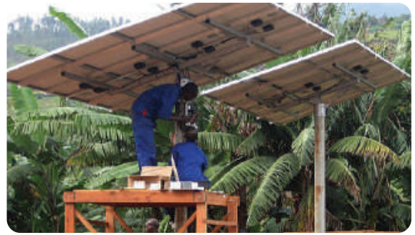
Fig 15.3 Technicians installing solar panels
