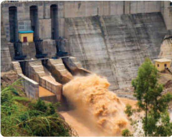
Fig 15.2 Nyabarongo hydropower plant in Muhanga district
