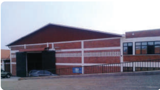
Fig 16.8 Warehouses for rent at the Kigali Free Trade Zone area
