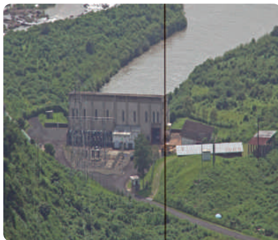
Fig 15.8 Hydroelectric power project on Rusizi River
