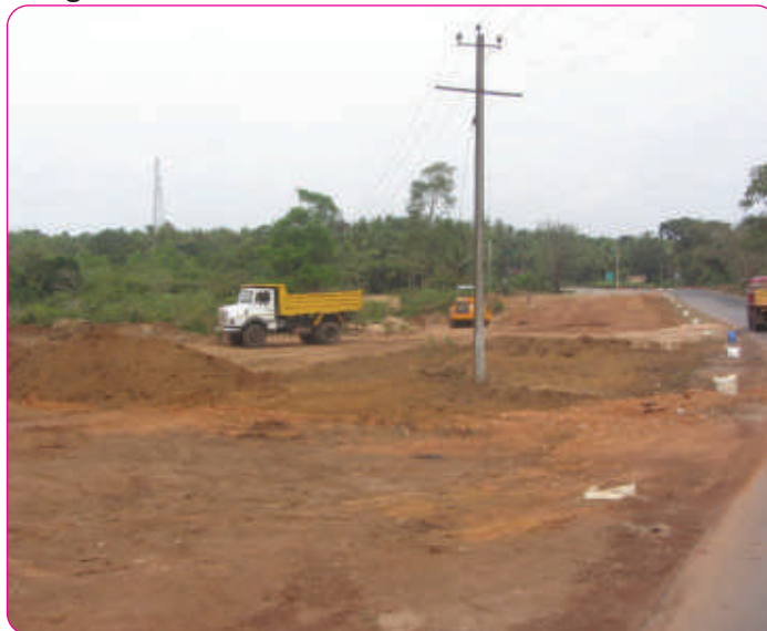
Fig 7.6 Levelling of land and clearing of vegetation for the construction of roads
